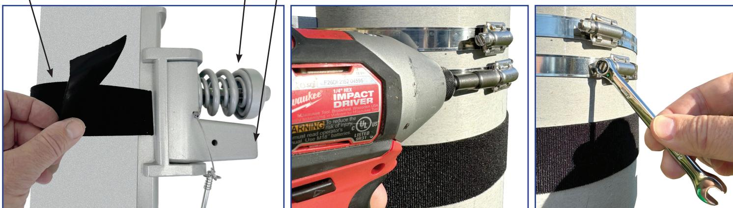
Pre-tighten hose clamps with cordless drill and 8mm~5/16" nut driver (included) and then finish tightening with included wrench.
